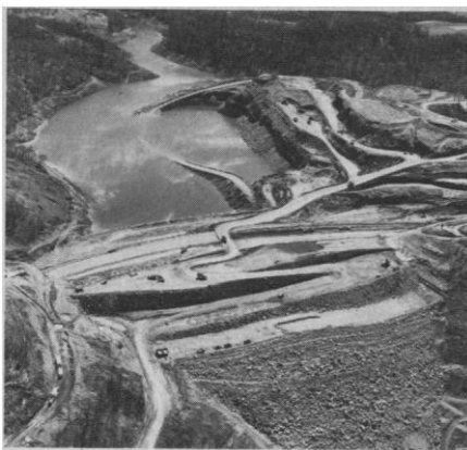
Fig. 1. Earth-fill dam being constructed across the mouth of Little Blue Run Valley, near Shippingport, Pennsylvania, to hold sludge that will be generated by lime scrubbers at the Bruce Mansfield Power Station. The completed dam will be an additional 150 feet in height and the valley will eventually be filled in with sludge to a length of more than 5 miles. [Source: Pennsylvania Power Co.]
