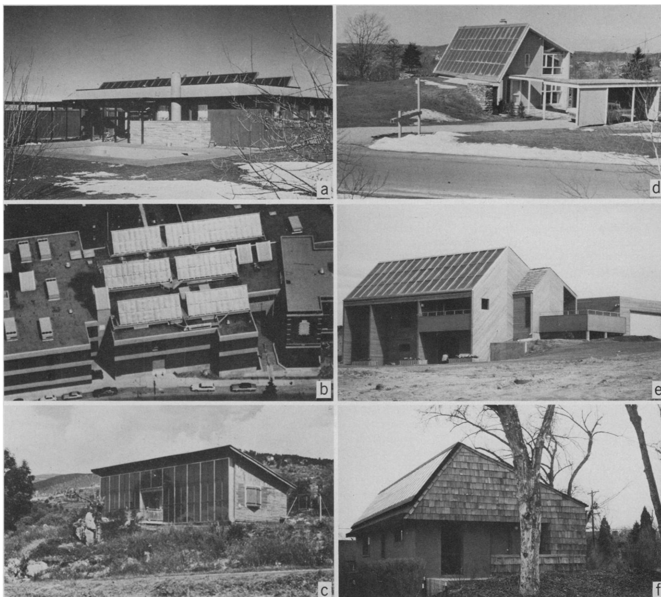
Fig. 1. Solar building architecture. (a) Löf home in Denver, Colorado. (b) Retrofitted collectors on school in Boston [photo courtesy of General Electric]. (c) Collector built into south wall of house of Odeillo, France. (d) MIT house IV, Massachusetts. (e) CSU house I, Fort Collins, Colorado. (f) Retrofitted house in Denver, designed by R. L. Crowther.
