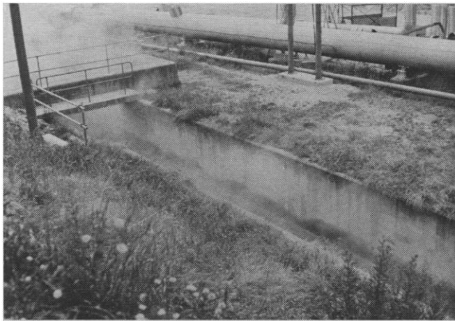
Fig. 5 (left). Steaming waste water, laden with dissolved silica and other minerals, flows through open concrete trenches to the Wairakei Stream and thence to the Waikato River. Fig. 6 (right). Steam mains from the Wairakei borefield pass under New Zealand Highway 1 to reach the power station. Large loops allow for thermal expansion and may ameliorate the effects of ground subsidence.
