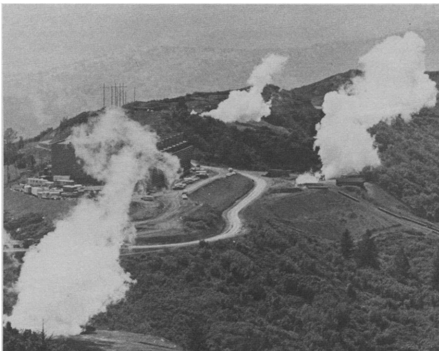
Two units of Pacific Gas and Electric's The Geysers plant in California. By 1977, there will be 15 units, with a total capacity of 908,000 kilowatts.
