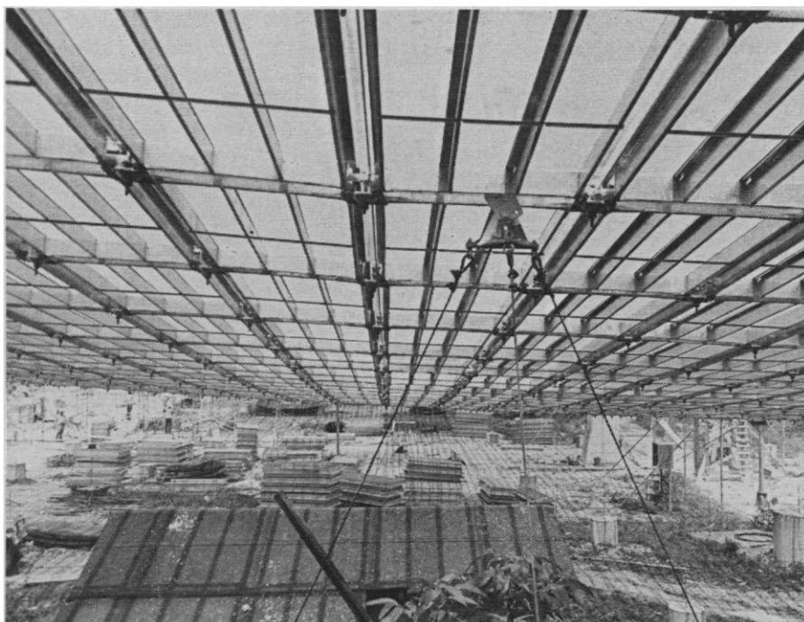
Fig. 2. Underside of the new reflector surface during placement of the panels. Note the cups fastening the common corners of four panels and the adjustment studs connecting to support cables.
