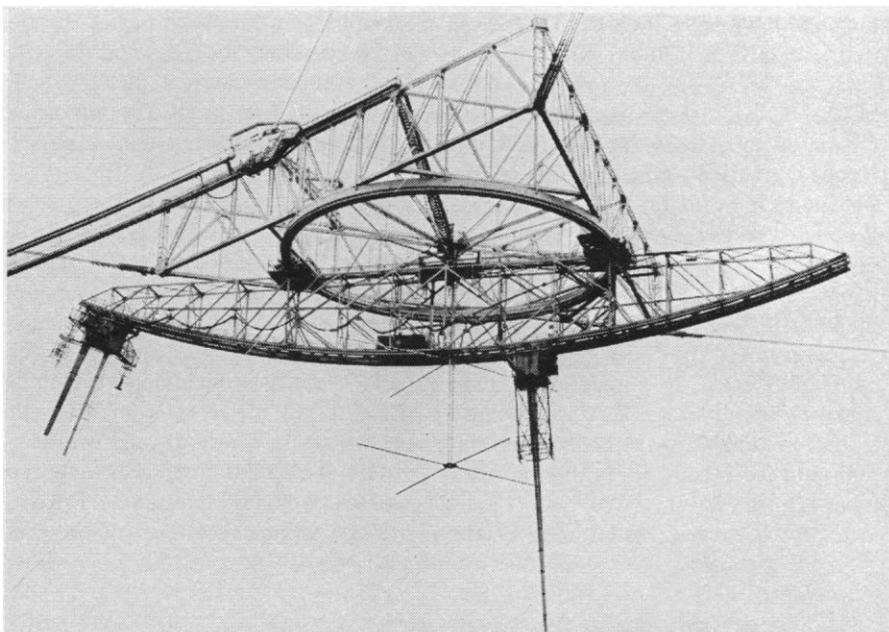
Fig. 5. Triangular support platform and rotatable feed arm truss suspended 150 m above the reflector. In this photograph, feeds mounted on the feed arm and carriage houses cover the range of frequencies from 6 to 611 Mhz, demonstrating the extreme versatility of the spherical reflector antenna.
