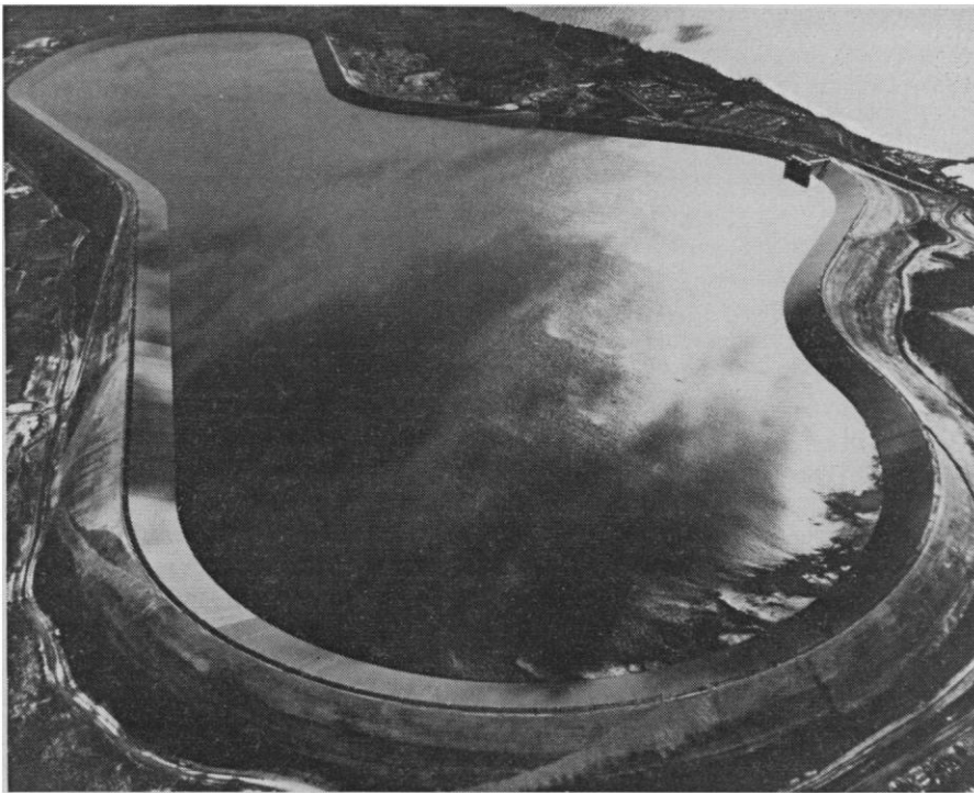
Fig. 1. The upper reservoir of the pumped hydroelectric storage plant near Luddington, Michigan. The reservoir embankment is 110 meters above Lake Michigan (upper right). The reservoir holds up to 102 million cubic meters of water.
