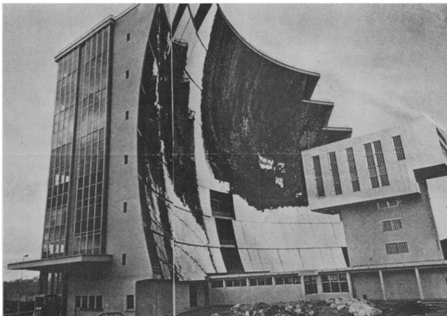
Fig. 1. The seven-story laboratory building at Odeillo, with the parabolic reflector mounted on its north wall and the target building to the right. [Courtesy of Life ]
