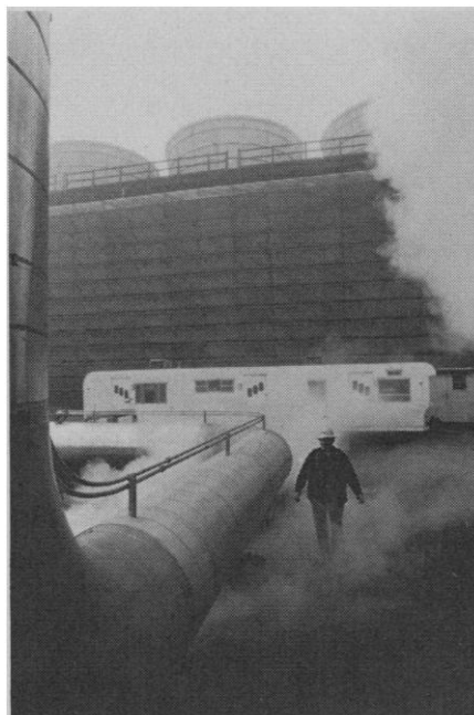
Fig. 3. Part of a 53,000-kilowatt generating unit at The Geysers geothermal power plant, Sonoma County, California. The big pipe is carrying steam to the turbine generators. Completion of this unit in 1973 brought the capacity of the plant up to 396,000 kilowatts. [Source: Pacific Gas and Electric Company, San Francisco]
