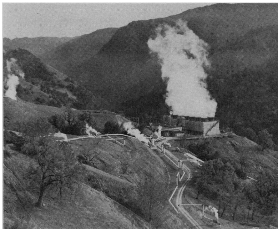
Fig. 2. Generating units at The Geysers geothermal power plant, Sonoma County, California. In the foreground are steam pipes with expansion loops. The loops allow the pipe to contract when the plant has to be shut down and to expand on start-up. The steam condensate rising from the row of five low stacks at the left marks the location of blowdown valves. When the plant has to be shut down, the steam escapes through these valves. The steam at the upper left comes from a natural fumarole. [Source: Pacific Gas and Electric Company, San Francisco]
