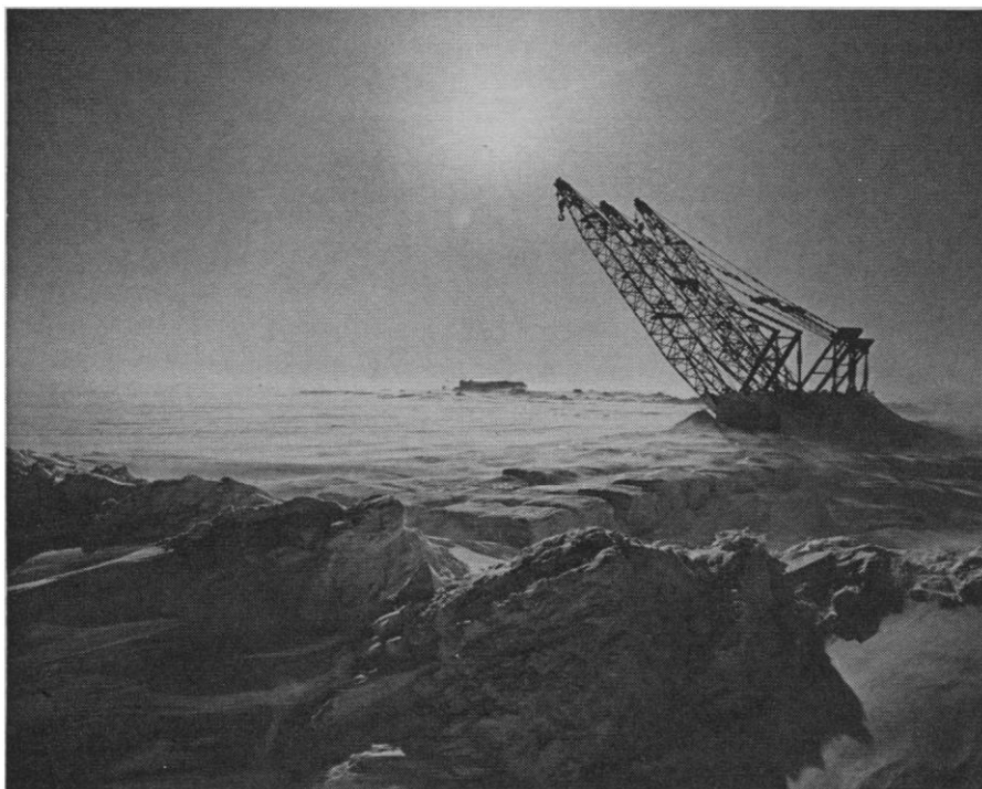
Cranes used in the unloading of barges which bring bulk supplies to Prudhoe Bay during the summer from Houston, Seattle, and other points. The ice moves off the Arctic coast for less than 2 months each summer and the barges have to slip through the moving ice and hurriedly deliver their supplies to avoid being frozen in for the winter. [Courtesy BP Alaska, Inc., Anchorage, Alaska]
