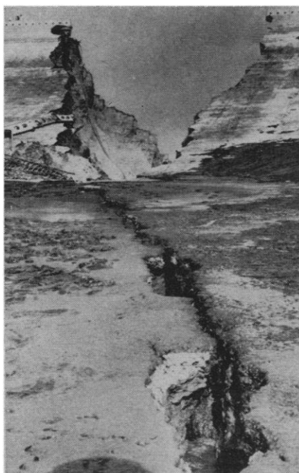
Fig. 1. Baldwin Hills Reservoir. Seepage through the ruptured reservoir lining (foreground) undermined and then breached the Baldwin Hills dam embankment (background). The relatively downward displacement of the ground surface to the left of the crack is clearly visible in the photograph. [Wide World Photo]
