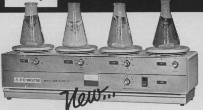
Thermolyne's new two and four place Multi-Stir Plates are designed for greater laboratory efficiency . . . no more reaching over hot surfaces . . . no more downtime because of belt problems . . . no more worry about heat control accuracy.
