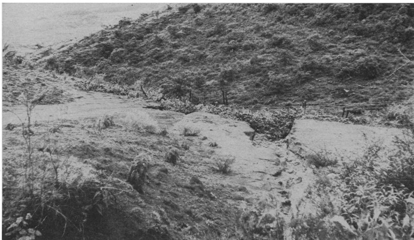
Fig. 10. Repair and stabilization of lama-bordo terrace at Yanhuitlan. Water and eroding soils are entrapped or slowed as they descend the natural drainage channels.
