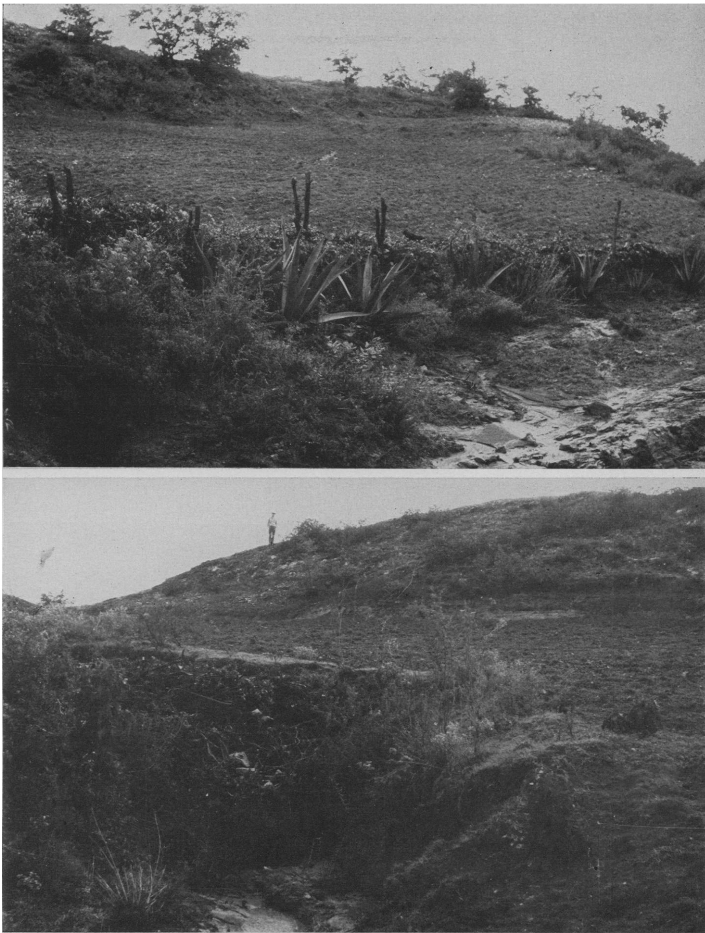
Fig. 9. Modern lama-bordo terraces at Yanhuitlan. Terraces are formed by accumulation of soil behind dikes of posts, brush, maguey plants, rubble, and stone. The structures are frequently reinforced with coursed masonry walls.
