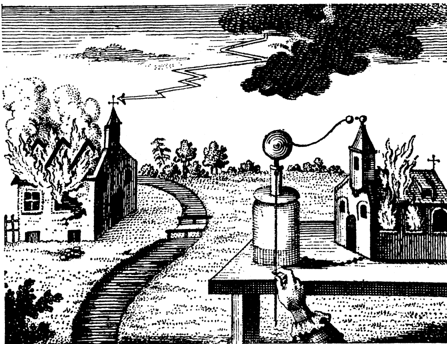
Equipment for demonstrating the virtues of lightning rods. In 1789 Harvard purchased from the Reverend John Prince a mahogany "thunder house" (similar to the model illustrated) 10 inches long and 8 high, with a lightning rod running up the gable. "Here was the lecturer's tour de force ! When the circuit was complete, an electrical charge passed through the lightning rod without harm to the house. But a spark supplied to a broken circuit ignited a quantity of gun powder inside the house, blowing off the roof and flattening the four walls amid a cloud of black smoke, fire, and general approbation from the students." [Reproduced in The Apparatus of Science at Harvard from Beck's Kurzer Entwurf der Lehre von der Elektrizität , 1787]
