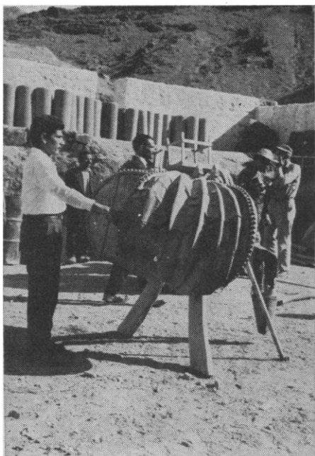
Fig. 7. Twin bellows for the smelting furnace of Fig. 6.
