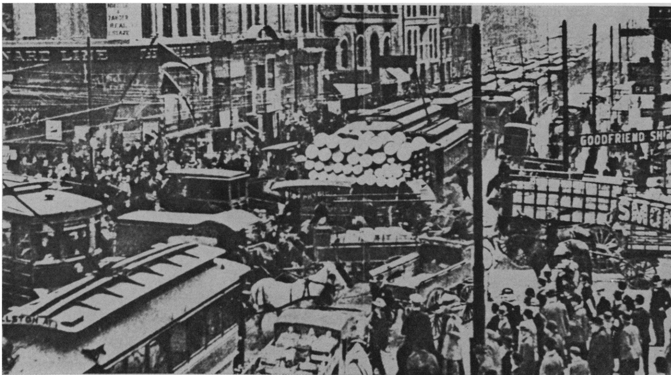
Fig. 1. Corner of Dearborn and Randolph Streets, Chicago, in 1910. [Bureau of Public Roads]
