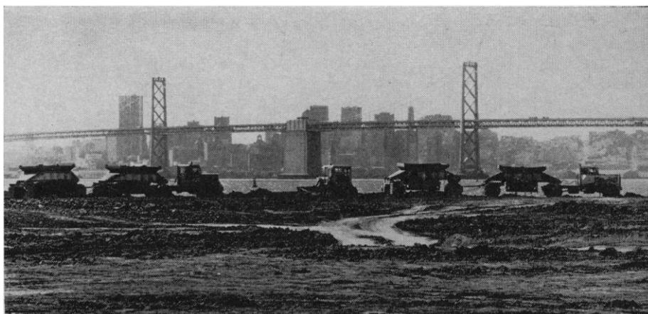
FILL-IN OPERATIONS: The Port of Oakland is creating this dock and warehouse site on San Francisco Bay over the objection of the California Fisheries and Game Department and private conservation groups. Most of the fill material is coming from the dredging of a trench for a rapid-transit tunnel. [Ron Partridge]
