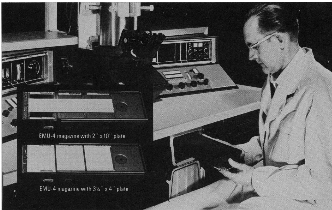
Front-loaded magazine holds 6 cassettes
