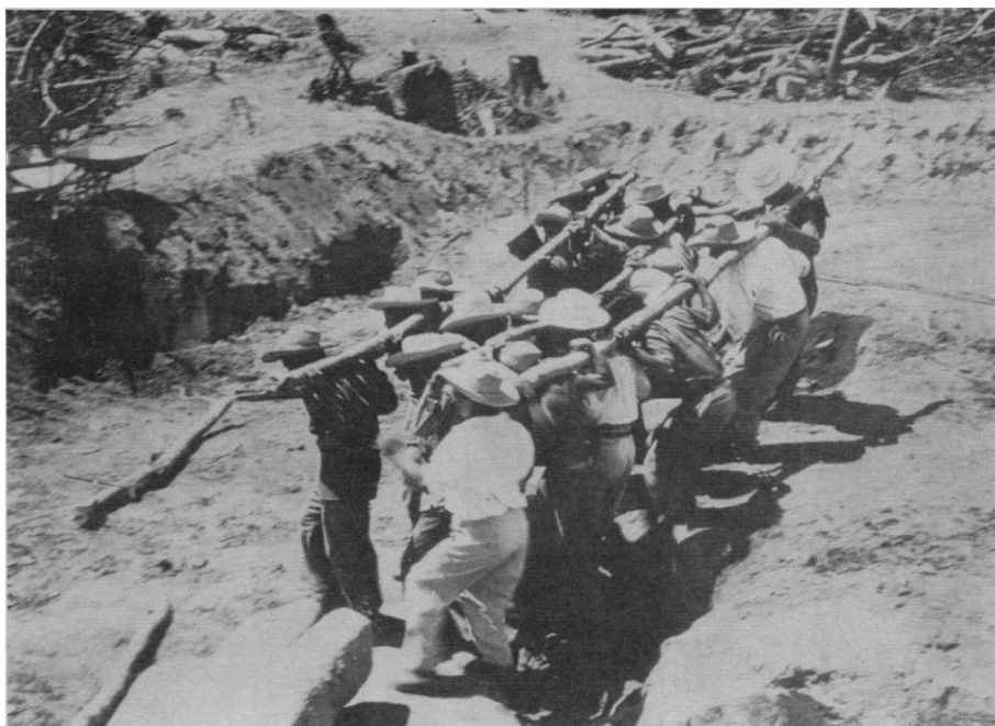
Fig. 6. Carrying a 1.5-ton stone column with poles and rope slings at La Venta, Mexico, in 1955. [Photo by author]
