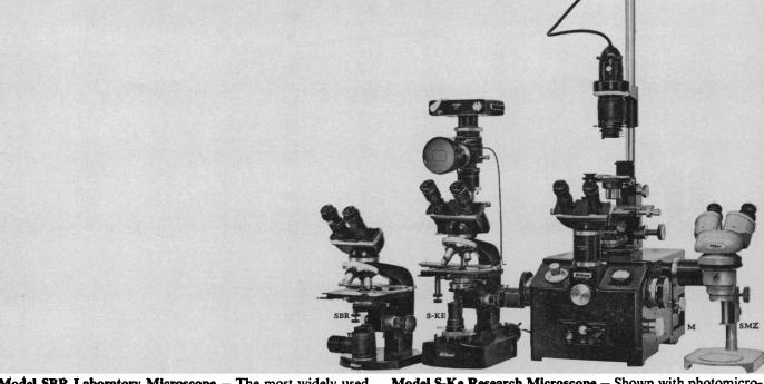
**Model SBR Laboratory Microscope** – The most widely used of the Nikon S series. A veritable workhorse for routine applications, yet easily adaptable to special requirements. Ready interchangeability of eyepiece body tubes, stages, condensers, oculars, objectives, etc., and a wide-variety of attachments and accessories, provide astonishing versatility.
