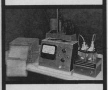
The YSI Model 53 Biological Oxygen Monitor System draws oxygen uptake or oxygen evolution curves in a few minutes. It records continuously, and useable information is available in only seconds after insertion of materials. It is stable, rugged, easy to use, easy to clean. Only a few minutes of technician training are required. The system costs \$1225.00 complete, except for a 100 MV recorder to draw the curves. May we tell you more about it?
