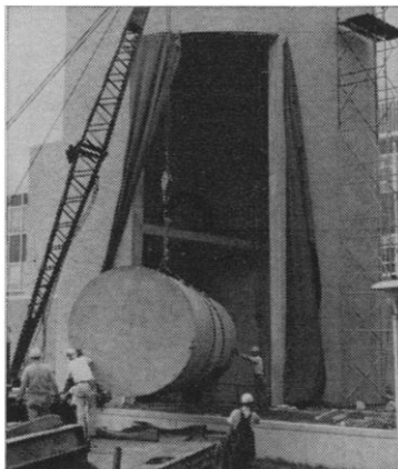
The University of Kentucky Van de Graaff is housed in a special cylindrical structure — part of the university's impressive new Chemistry-Physics building.
