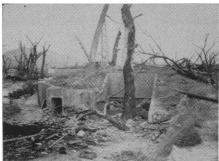
Fig. 3 (left). Chugoku Army Headquarters (750 m from ground zero). Underground communications trench. Entrance at left. (AFIP Neg. HB 321.) Fig. 4 (right). Chugoku Army Headquarters (750 m from ground zero). Underground communications trench. Open metal port. This is a view looking away from the center of the explosion, with which the optical axis of the camera is in line. (Reprinted by permission from A. W. Oughterson and S. Warren, Medical Effects of the Atomic Bomb in Japan (McGraw-Hill, New York, 1956), p. 61.) (AFIP Neg. HB 320.)
