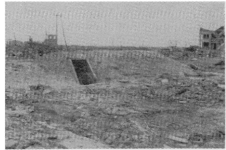
Fig. 1. "Hiroshima. Typical, part below ground, earth-covered, timber framed shelter 300 yds. from the centre of damage, which is to the right. In common with similar but fully sunk shelters, none appeared to have been structurally damaged by the blast. Exposed woodwork was liable to 'flashburn'. Internal blast probably threw the occupants about, and gamma rays may have caused casualties." (Reprinted by permission from Report of the British Mission to Japan (3) and the Imperial War Museum, London.)
