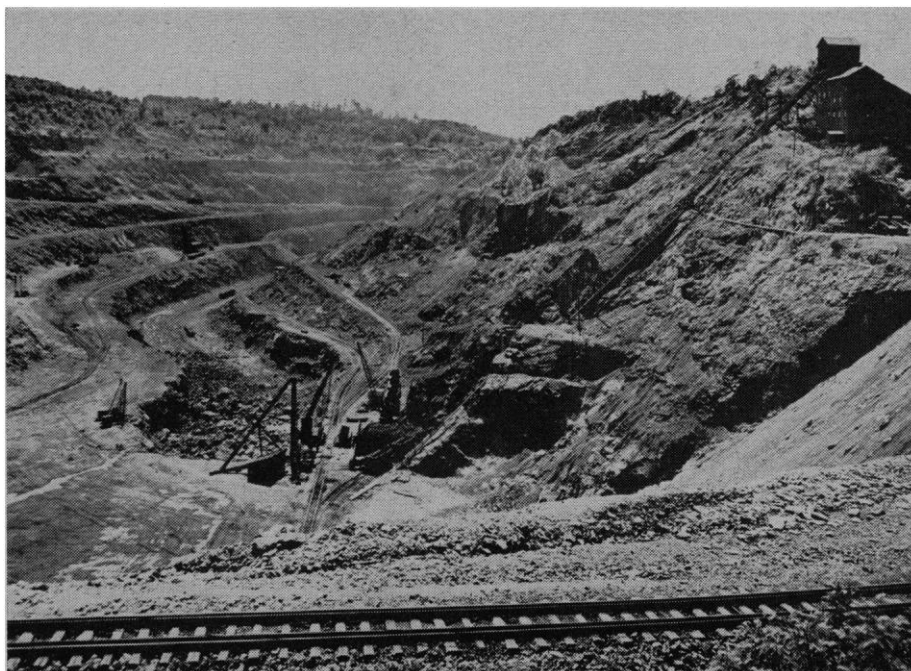
Mining ore by the open-pit method at the Cornwall, Pa., mine of the Bethlehem Steel Co.
