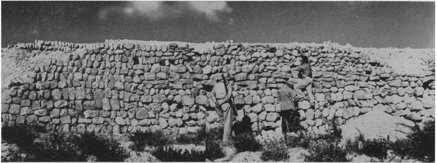
Fig. 10 (above). A diversion canal wall of the Nahal Lavan system. Note the different stages of construction. The foundations are about 2 meters below the present soil surface. Fig. 11 (bottom of page). A large spillway with a crest length sufficient to allow passage of large floods.
