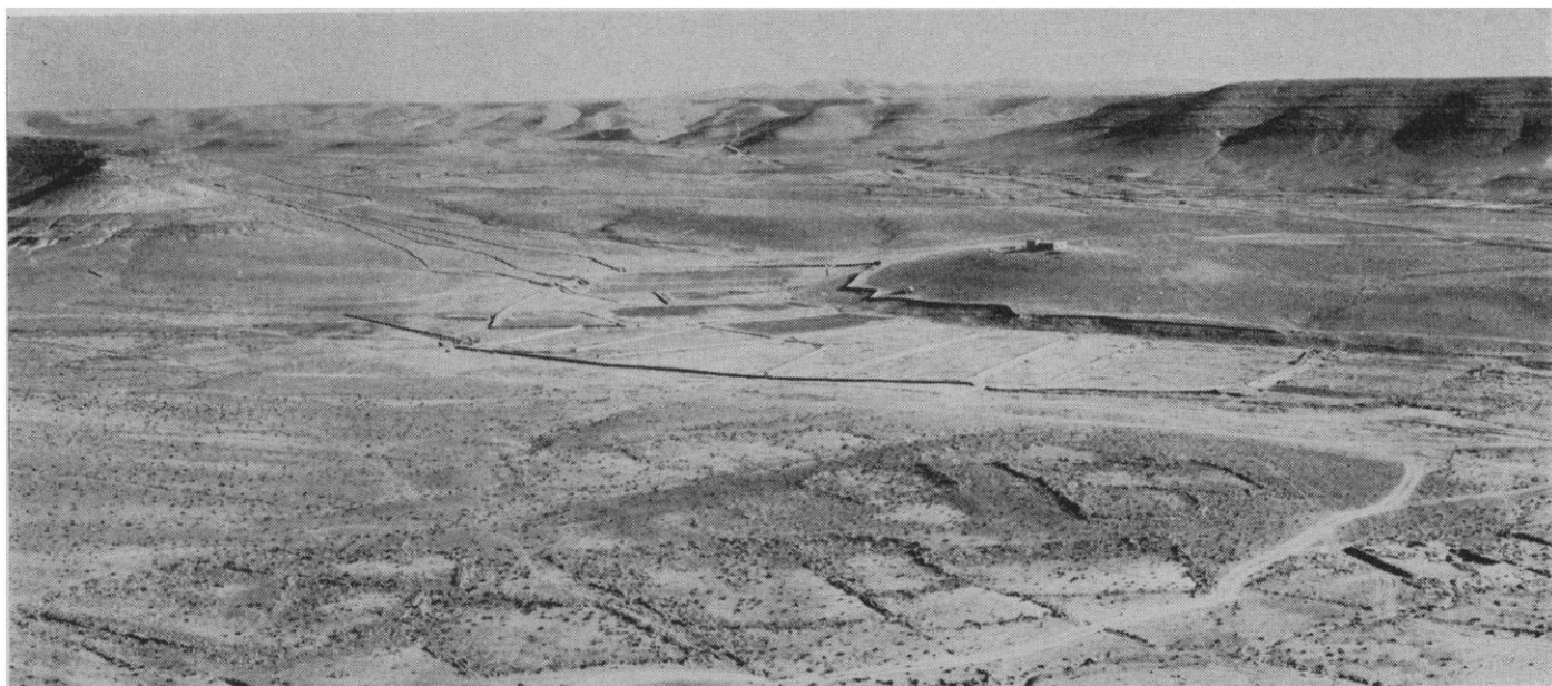
Fig. 15. The reconstructed ancient farm near Avdat. Note the farmhouse on the hill. The reconstructed conduits leading runoff from the small watersheds may be seen in the background.
