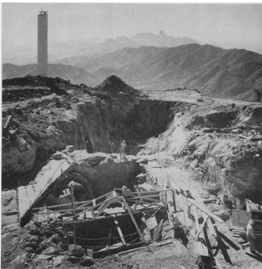
Site of the solar telescope at Kitt Peak National Observatory in the Quinlan Mountains of Arizona. The large hole in the foreground will contain the observing room. The tower at left contains meteorological instruments used in the site survey. Famous Baboquivari Peak in the distant background is the sacred mountain of the Papago Indians, on whose reservation the national observatory is located.
