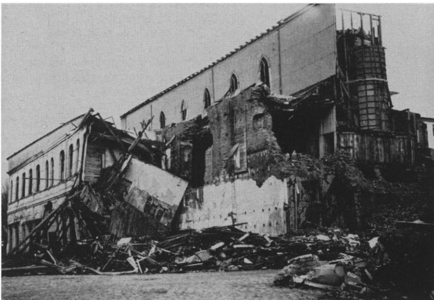
Fig. 9 (left). Collapse of a composite wood-frame and adobe building in Valdivia. Fig. 10 (right). Failure of the supporting members of an elevated water tank in Rio Negro.
