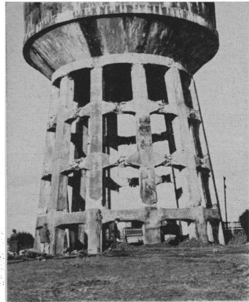
Fig. 9 (left). Collapse of a composite wood-frame and adobe building in Valdivia. Fig. 10 (right). Failure of the supporting members of an elevated water tank in Rio Negro.
