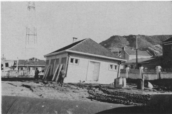
Fig. 7 (left). Settlement at the naval base, Puerto Montt. Fig. 8 (right). Relative horizontal movement of two parts of a building near the naval base, Puerto Montt.
