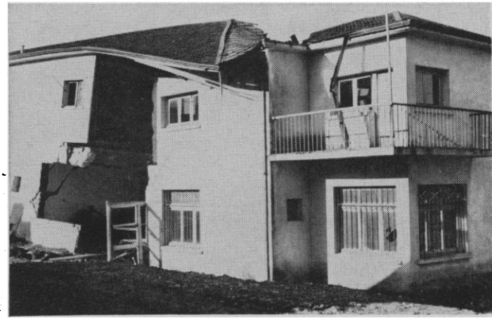
Fig. 7 (left). Settlement at the naval base, Puerto Montt. Fig. 8 (right). Relative horizontal movement of two parts of a building near the naval base, Puerto Montt.
