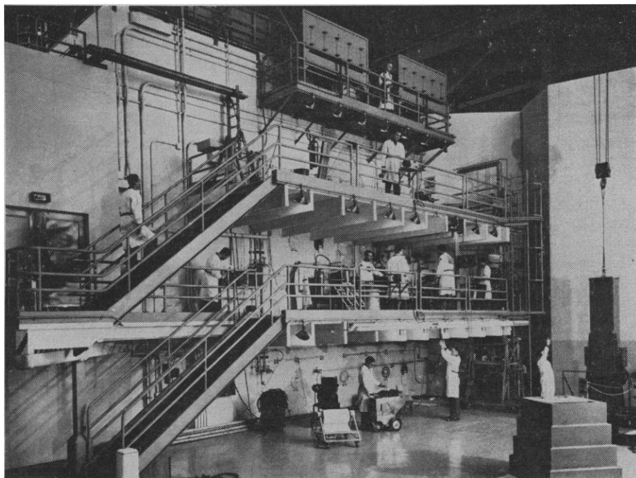
The west face of the Brookhaven Graphite Research Reactor at the Brookhaven National Laboratory. On the first balcony, physicists and chemists are measuring the energy from beams emerging from the reactor, while on the ground floor and on the second balcony, health physicists are monitoring the ports to check for possible radiation leaks. This reactor is one of the four which the United States has offered to place under the proposed safeguards system of the International Atomic Energy Agency. The Brookhaven National Laboratory is one of the Atomic Energy Commission's principal research facilities.
