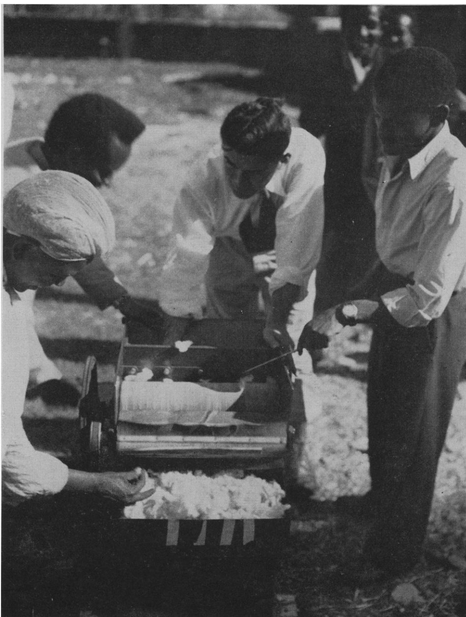
An FAO specialist in cotton production demonstrates a light ginning machine to his Ethiopian colleagues. Though not a supply agency, FAO does provide limited amounts of equipment and supplies as a part of its technical assistance work.
