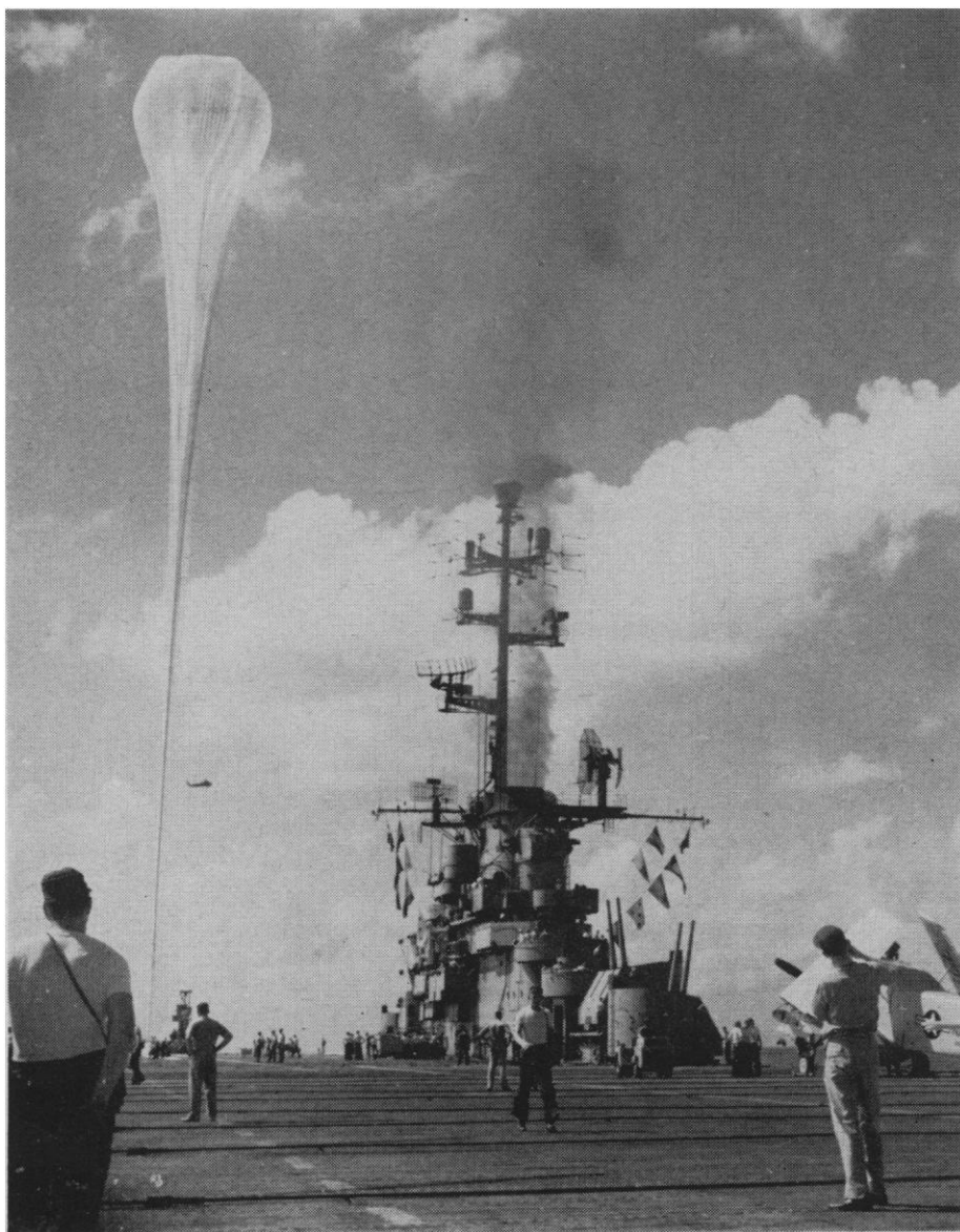
Skyhook Bravo Re-Fly just before launching. With inflation tubes tied off and dangling, the balloon stands nearly 500 feet above the deck of the U.S.S. Valley Forge .
