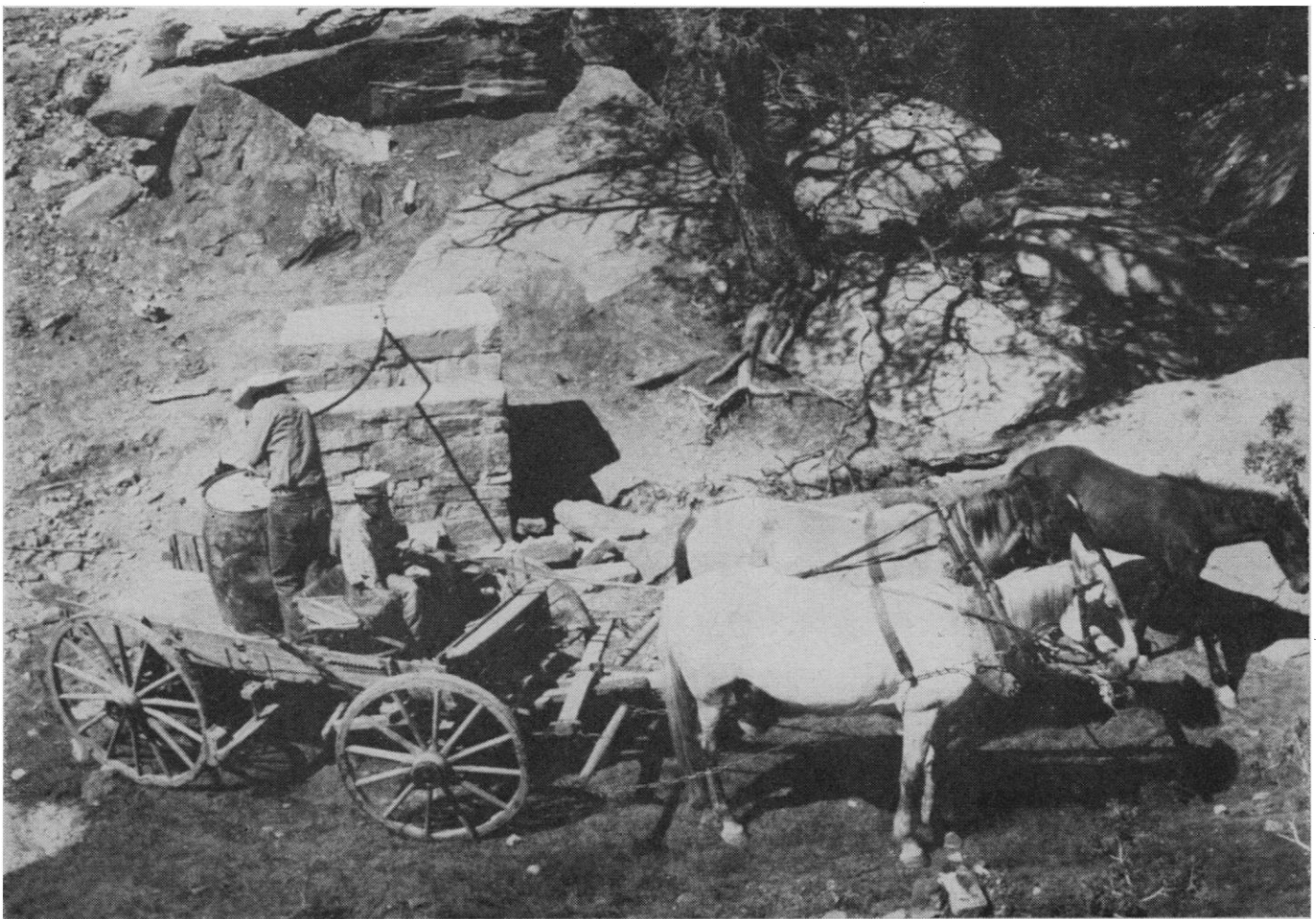
Filling the camp water barrel by hose from a protected spring. The water may have to be hauled from 2 to 10 miles to the individual homes. The water is uncontaminated at its source but may easily become contaminated by necessary handling and the use of a communal dipper in the hogan. An extensive community program has been started, with tribal funds, to erect structures to protect the springs, such as that seen here, and to restore "sanded" wells. The unbroken colt is simply accompanying its mother while she works and is one more feeder on the overgrazed range. [James Bosch, Window Rock, Ariz.]
