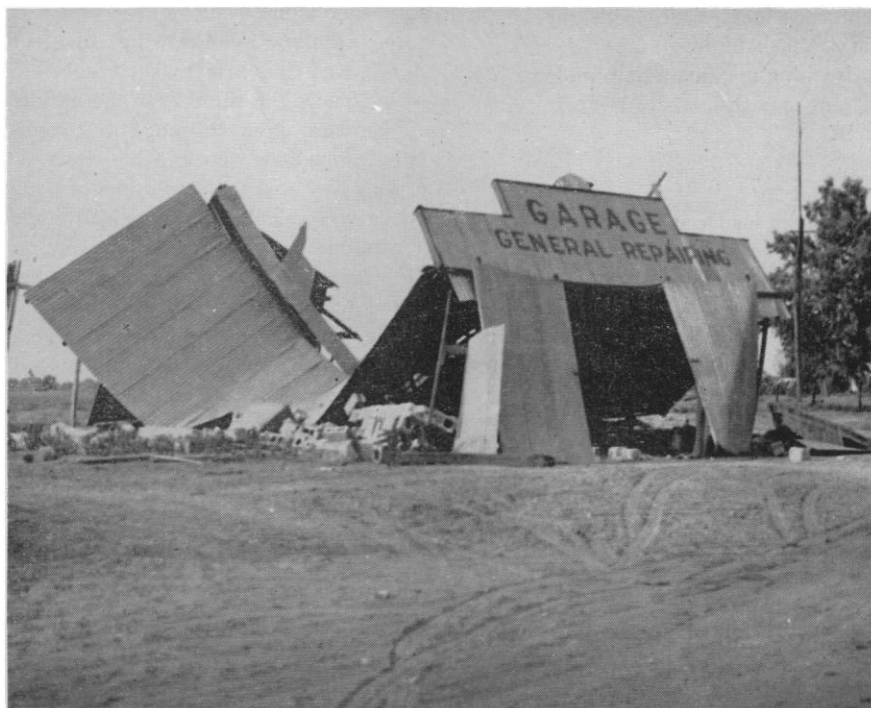
Damage due to shaking, near Meloland, California, May 1940. [Photograph by J. P. Buwalda. From Elementary Seismology ]
