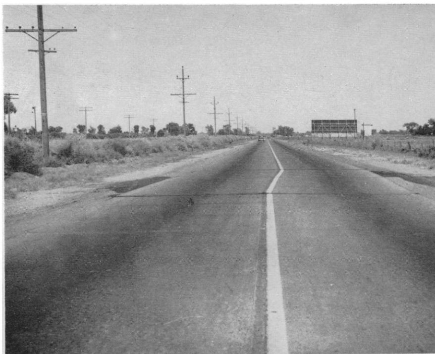
Highway offset horizontally by faulting, as indicated by the painted center strip, in Imperial Valley, near Meloland, California, May 1940. [Photograph by J. P. Buwalda. From Elementary Seismology ]
