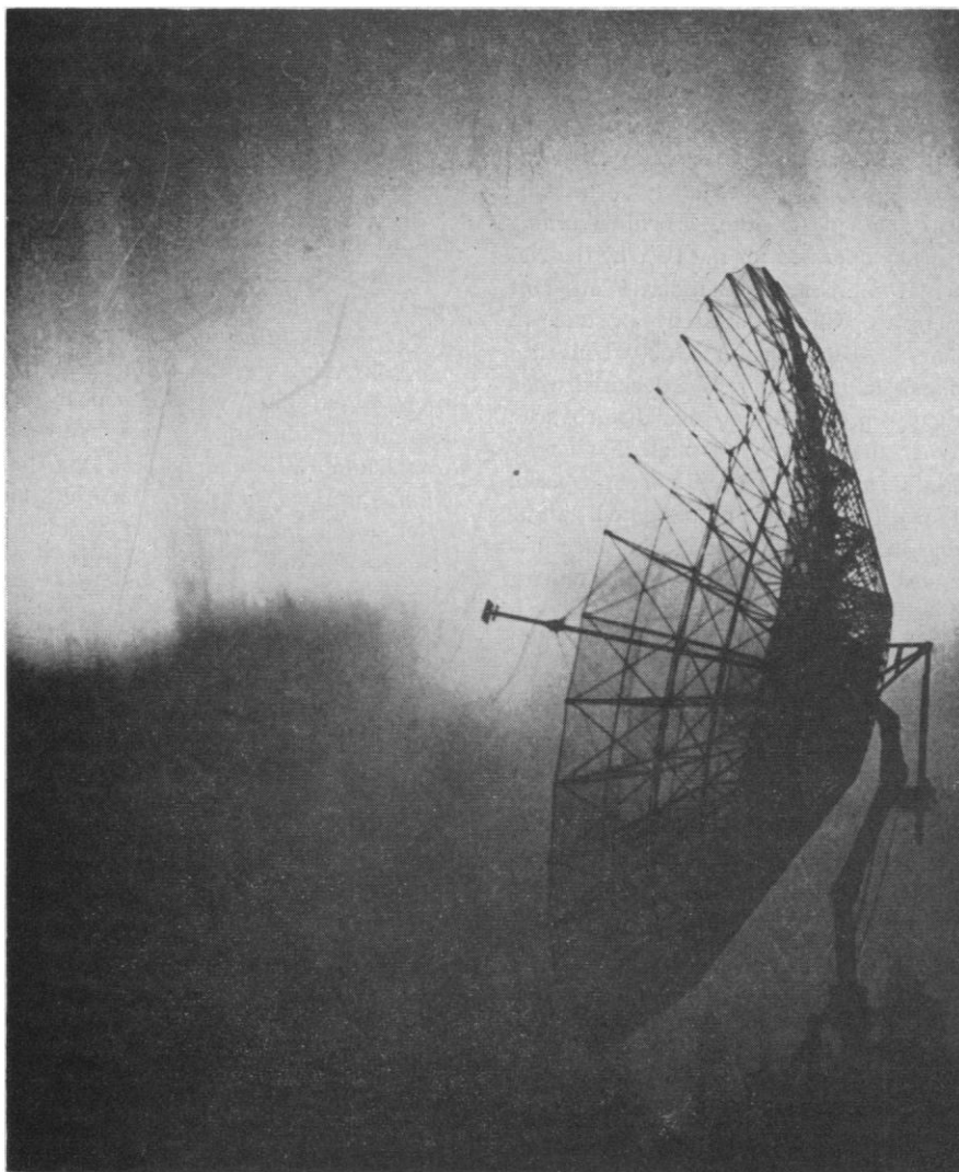
Parabolic antenna, with aurora borealis in the sky, used at College, Alaska, to study radio noise and radio wave reflections from the aurora. [Stanford Research Institute]
