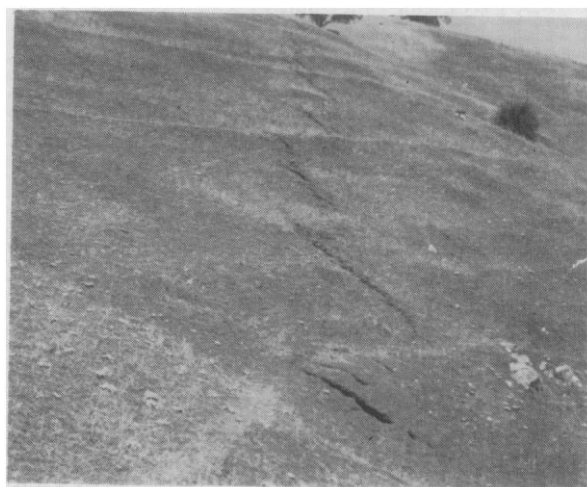
FIG. 4. Typical en échelon cracks, indicating left-hand horizontal shearing movement. Near Tunnel 5 of Southern Pacific Railroad.
