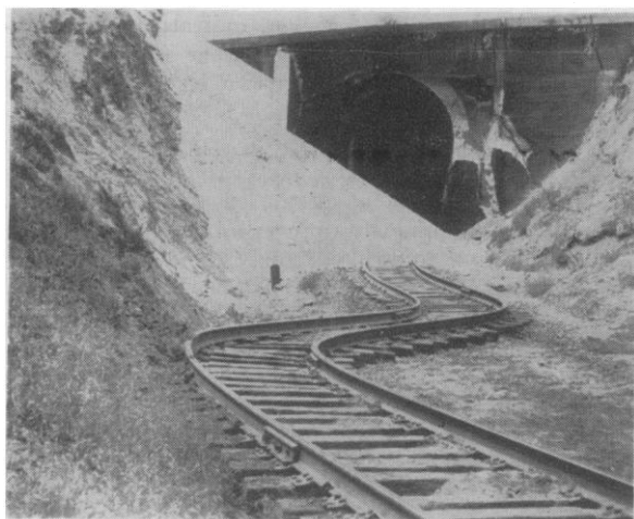
FIG. 7. View north toward the south end of Tunnel 3 of the Southern Pacific Railroad, showing part of damage to tunnel where one of the long cracks crossed the bore near its portal at a large angle. Also shows sharp kinking and presumed shortening of track by some eight feet, part of which occurs beyond white waste pile within tunnel.
