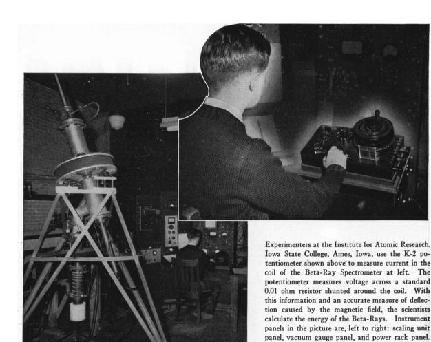
Measure Current Precisely with K-2 Potentiometers
