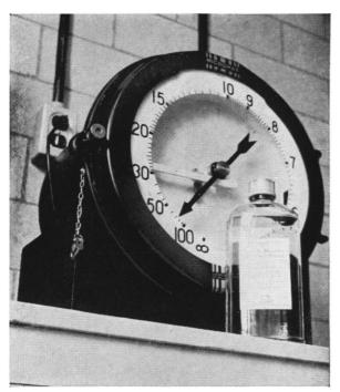
Upjohn Co., Kalamazoo, Mich., use this Micromax Recorder to show the constant purity of the sterile, doubledistilled, pyrogen-free water which is one of their products. Shown below is the equipment's metal-boxed conductivity-cell assembly.
