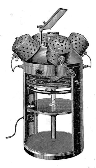
THIS instrument for the first time supplies adequate illumination by means of incandescent bulbs for the projection of large opaque objects. The area illuminated is 20 x 20 cm.
