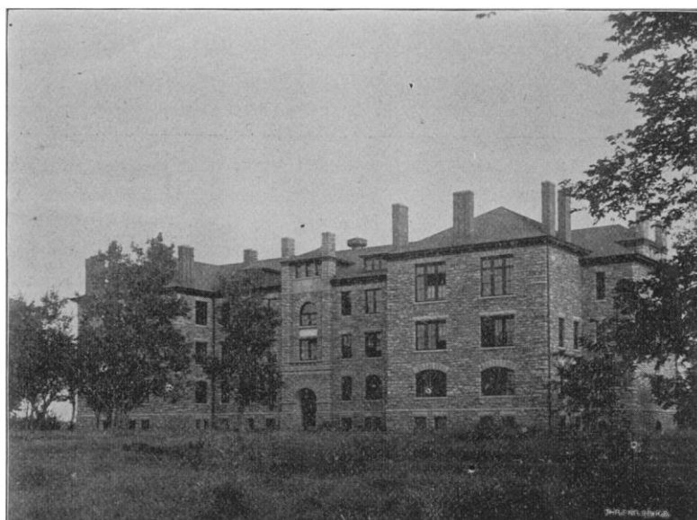
Chemical Laboratories. South Front.
