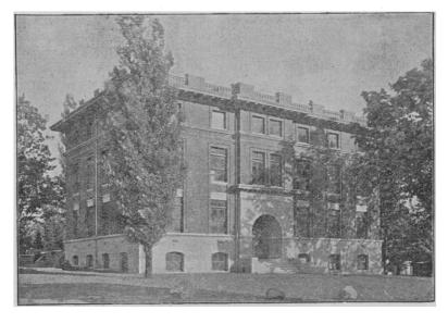
The cut of the exterior and the floor plans here presented will give the reader a general idea of the structure. The general form of a building that would best suit the requirements of the various departments was found to be a rectangle,  $52\times88$  feet. This is divided into two parts in each story by a hall 13 feet in width. This provides a wide, recessed entrance on both sides of the building.
