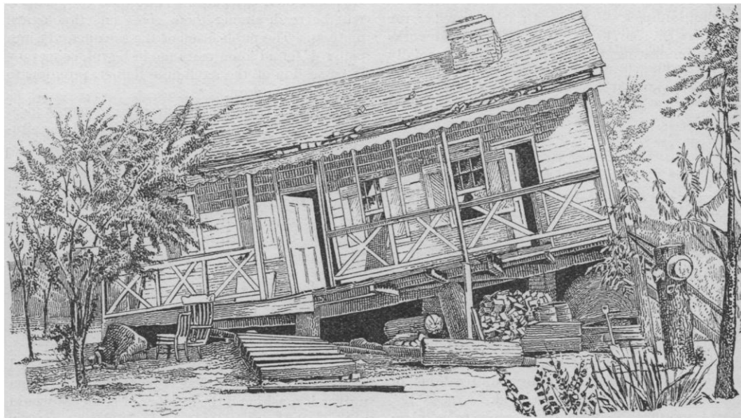
HOUSE IN LINCOLNVILLE, SHOWING CHIMNEY-BASE CRUSHED BY UPWARD MOVEMENT OF THE EARTH.
