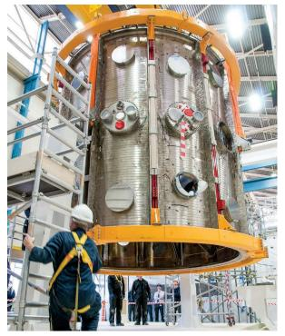
Engineers lift out MAST's vacuum vessel for modifications during the £30 million upgrade.
