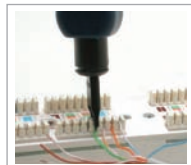
Punch and cut cable terminals
