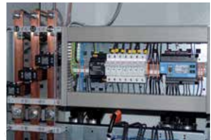
Fig.: Capacitor monitoring in a PFC system
