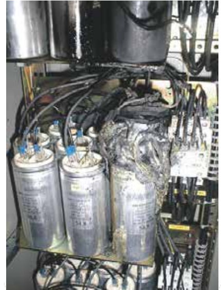
Fig.: Capacitors destroyed due to harmonics
