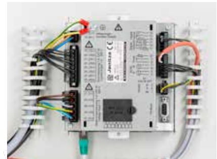
Fig.: UMG 512-PRO for monitoring the EN50160
