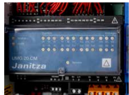
Fig.: UMG 20CM for recording the load flows
