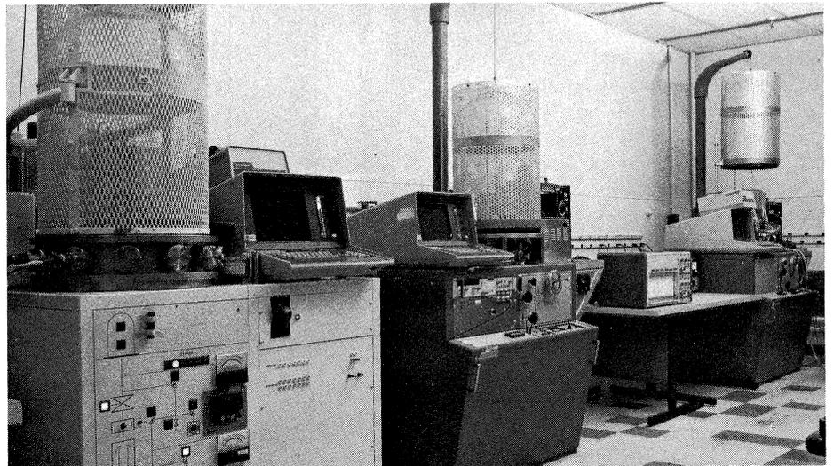
Fig. 3. Three of the four automated test stations. In the two stations on the left, clock assemblies are being tested under the bell jar in a simulated space atmosphere. The right station bell jar is about to be lowered to the base plate on the vacuum stand.
