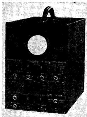
*On the right is shown the panel view of the Dayrad Series 65 Oscilloscope. All the controls are on the front panel with the exception of the horizontal and vertical spot positioning controls, which are on the side of the cabinet. A 1000-cycle, frequency-modulated oscillator is incorporated in the unit.*
