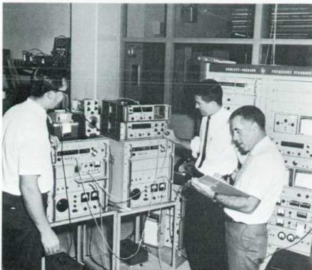
*-hp- engineers Lee Bodily, Dexter Harthe, and Ron Hyatt calibrate flying clocks with -hp- house standard prior to globe-girdling trip.*
