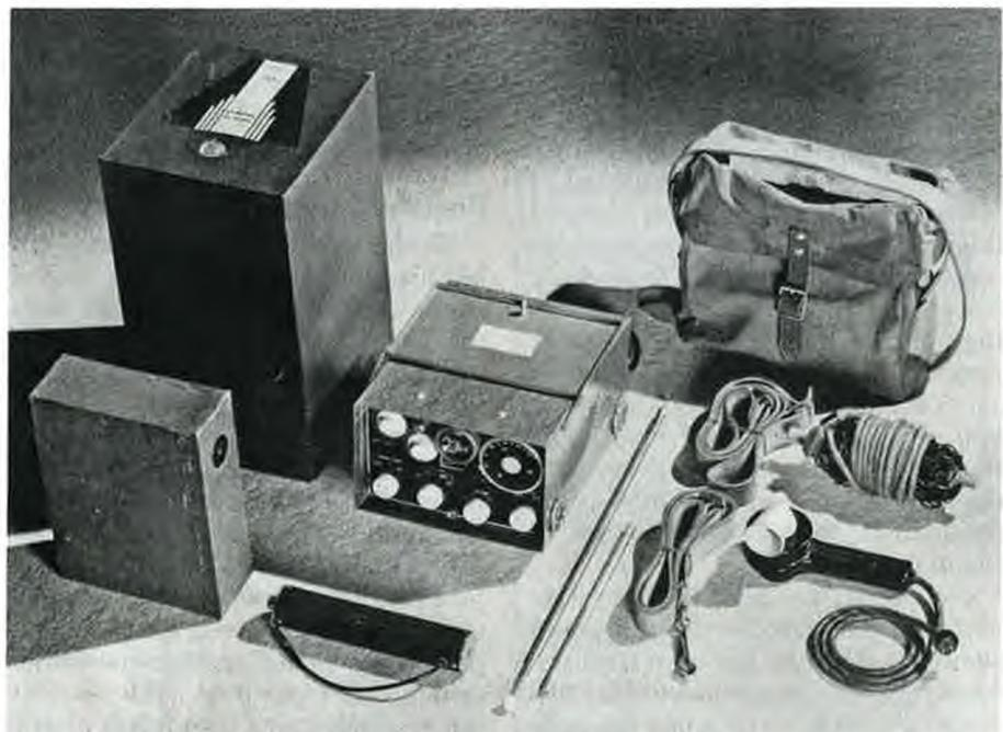
Taken from the handbook, this photo shows the TRP-1 transceiver (centre) complete with all its accessories, including batteries, antennas and the microphone. The large "camp" battery at top left was optional
