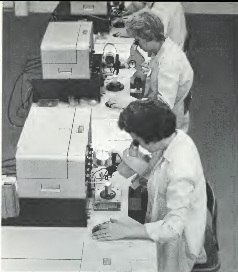
**TESTING** — Each Transitron integrated circuit is tested on automatic, high-speed, multi-parameter test systems. These test systems, which were designed and constructed at Transitron, also include a punched paper tape output of test results for data logging and computer analysis of test data.
