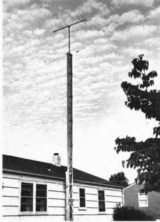
Fig. 3 — While guys are not normally required for the homemade tower, they provide an extra measure of protection against high winds. An inverted V can serve here as two of the guy lines.
