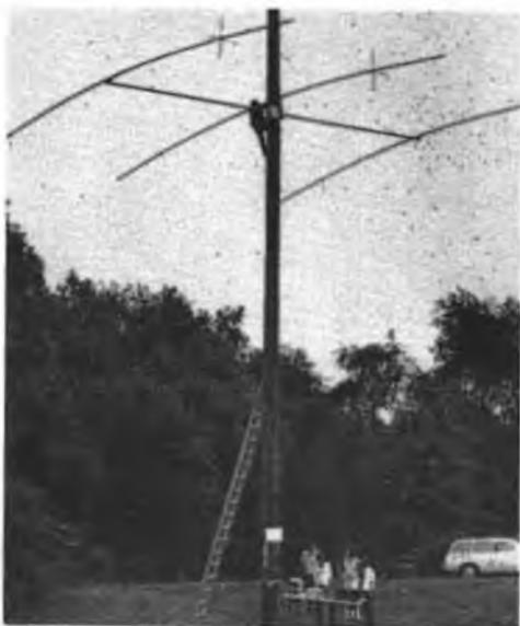
Fig. 1 — The short 40-meter Yagi resembles a large 20-meter system.
